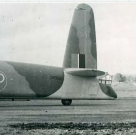
Windsor NK136 outside Vickers' hangar at Wisley in 1945 after gaining its rear-firing twin 20mm Hispano cannon
