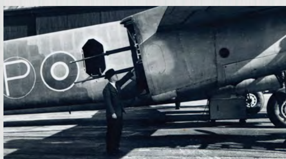
ABOVE Vicker's design engineer, Sammy Walsh, inspects NK136's rear-firing cannon. The only example to receive its defensive armament, the manufacturer gave the airframe the new designation Type 461
