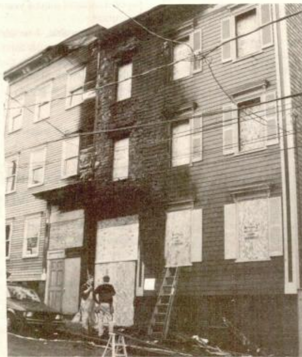
THE TASK of boarding up the burned-out houses at 84-88 Bartlett St. was undertaken on Monday afternoon. Renovations to the house at the left were almost complete following a March 15, 1990 blaze.
