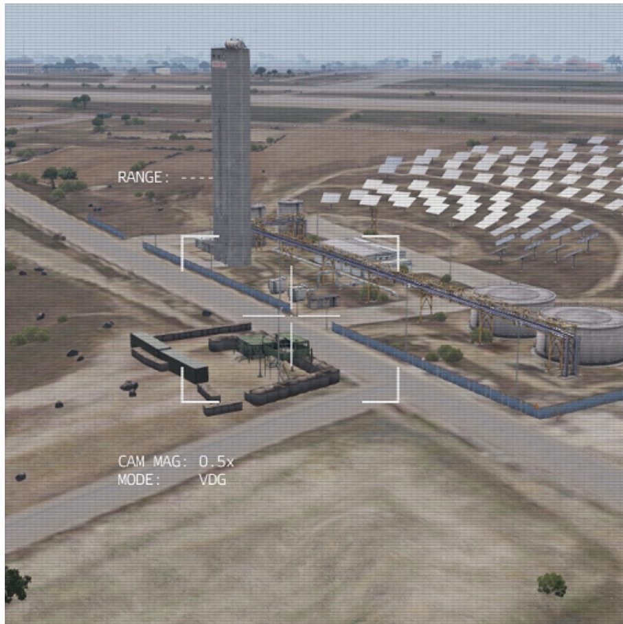
Altis Solar Power Plant
