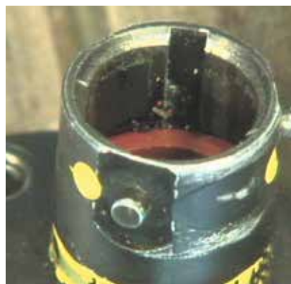
Figure 4: Vibration and the stress of high loaded cables have worn away this connector's zinc plating
