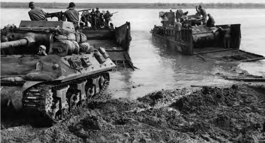
ABOVE: Two M-36 tank destroyers from a U.S. Ninth Army unit roll onto U.S. Navy LCMs (Landing Craft, Mechanized) in preparation for an assault crossing. Such large craft had to be transported to the river on tank-retriever trailers. BELOW: A rare color photograph shows 79th Infantry Division troops preparing to cross the river at Orsoy, Germany, north of Duisburg, March 10, 1945. The boats in the foreground are bridge pontoons. OPPOSITE: A crane lifts an LCVP (Landing Craft, Vehicle and Personnel) into position prior to the Rhine crossing.
