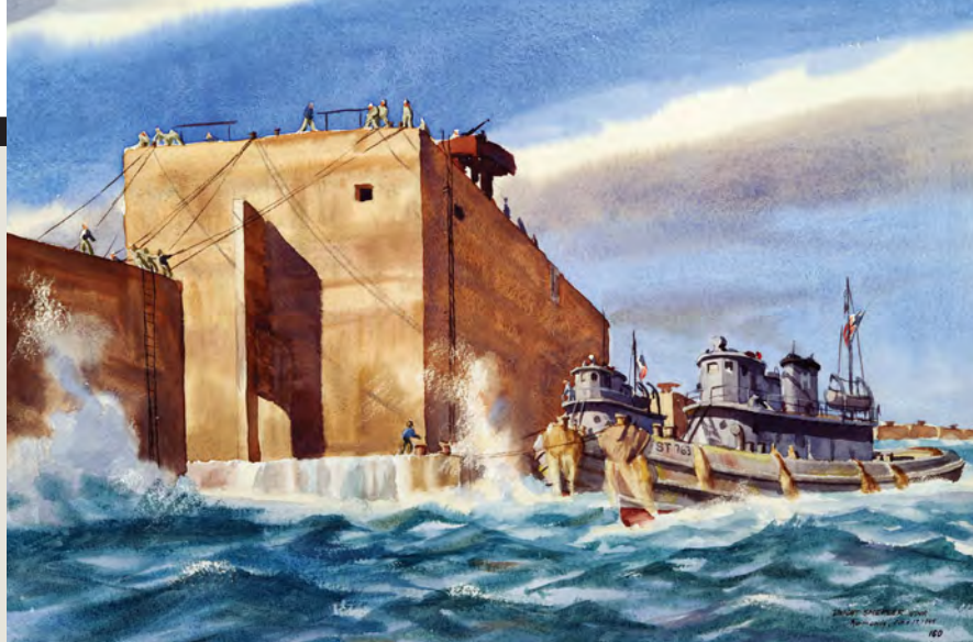
ABOVE: The Seabees weren't just in the Pacific. Here a section of the artificial Mulberry harbor, built in England, is towed across the Channel to Normandy. Seabee crews rode the Mulberry across the Channel and opened the sea valves to sink the concrete structures at Omaha Beach. OPPOSITE: Seabees have “married” a pontoon causeway to an LST to offload cargo from ship to shore on an unnamed island.
