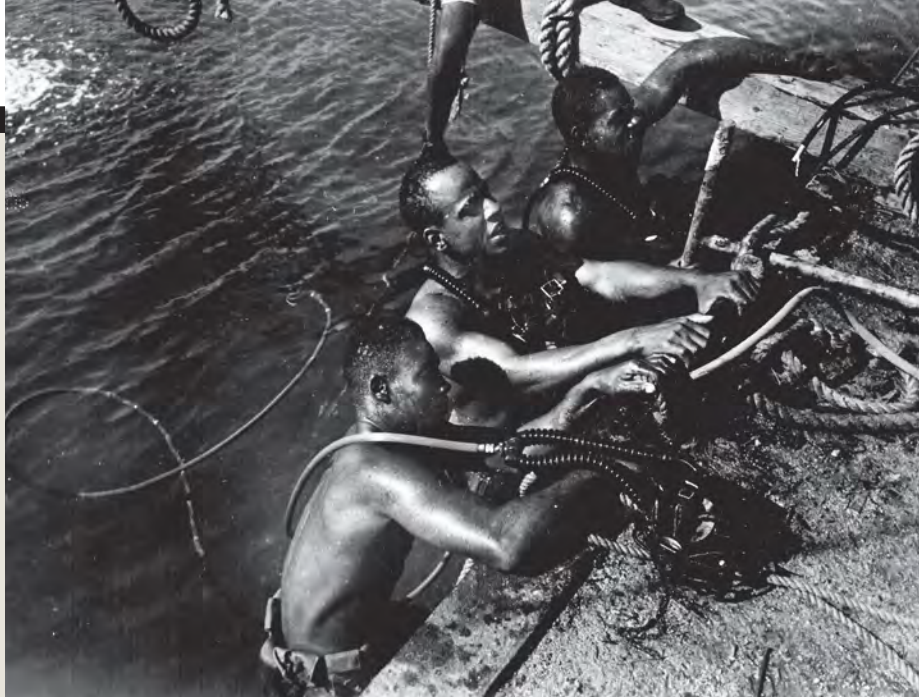
ABOVE: African American divers of the 34th Seabee Battalion—a nonsegregated unit—work on the marine railway at Gavuta in the Solomon Islands, 1944. At the height of the war, there were more than 12,000 black Seabees. OPPOSITE: Seabees lay Marston mats during runway construction on Bougainville. Developed before World War II, the Marston Mat consisted of perforated steel planking strips primarily used for the rapid construction of temporary runways and landing strips.
