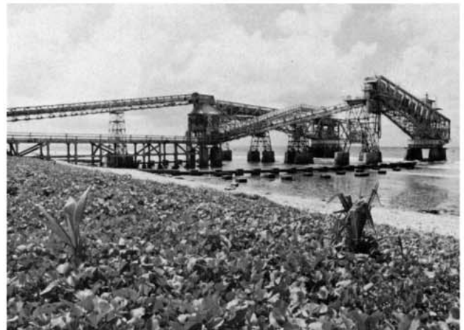
Though needed to carry the phosphate across the shallow reef to ships anchored offshore, it was not repaired until 1948.
