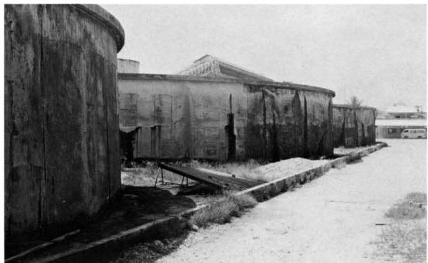
The oil storage tanks were replaced by new ones during the post-war reconstruction.
