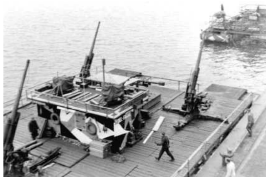
■ A heavy flak Siebel ferry with the 4-metre rangefinder placed ahead of the wheelhouse which is being fitted-out. Note the transport ferry having its structure put together alongside the dock. These ferries were modular, easy to move by rail and extremely versatile.
