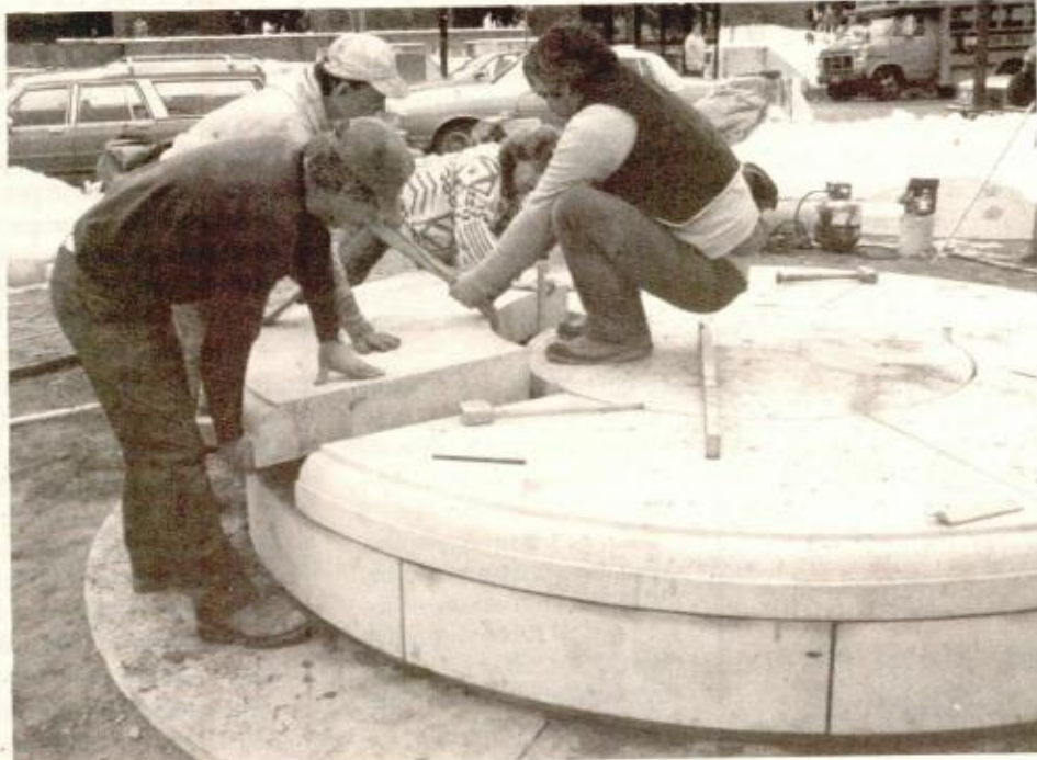
WORKERS INSTALL granite slabs which form parts of the sundial.
