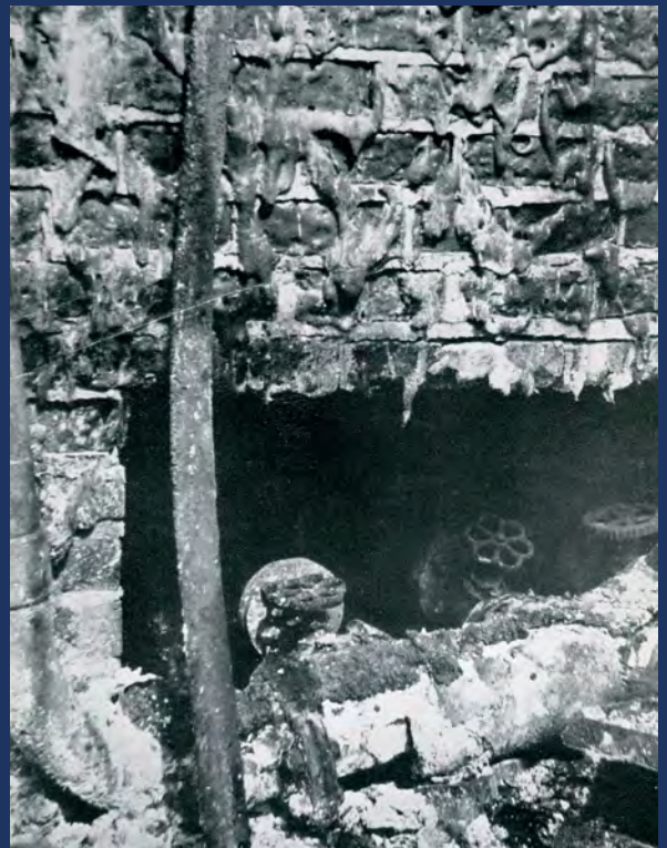
BELOW: The fires were so intense at Purfleet, even the bricks of the surrounding bund wall began to melt [PETROLEUM AT WAR, 1946]
