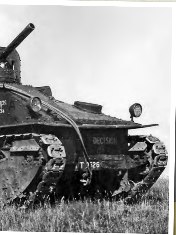
Above: Photographed at Vickers, Newcastle, one of the tanks supplied to Russia. The turret is identical to the one supplied to Australia but it's running on a Mark IIA hull. Only this one, we think, carried a three-pounder gun.
