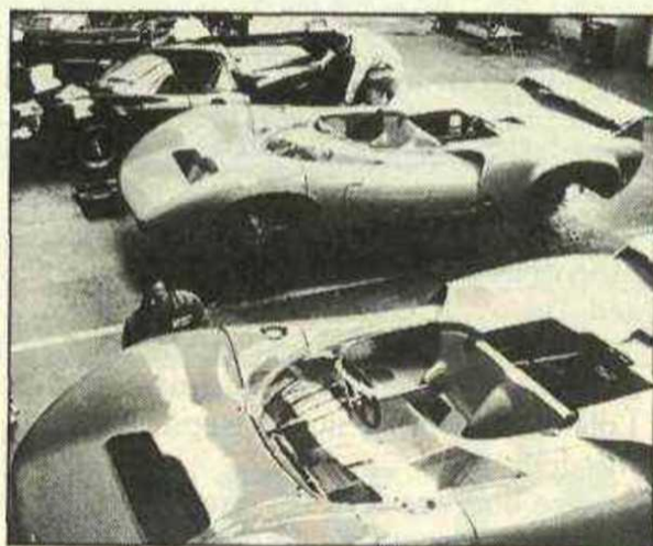
Two of the four MkIII B spyders under construction at Slough for Roger Penske.
