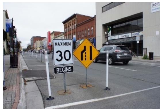
Figure 31. Gateway signage and a reduced number of travel lanes are valuable elements for reducing vehicle speed.
