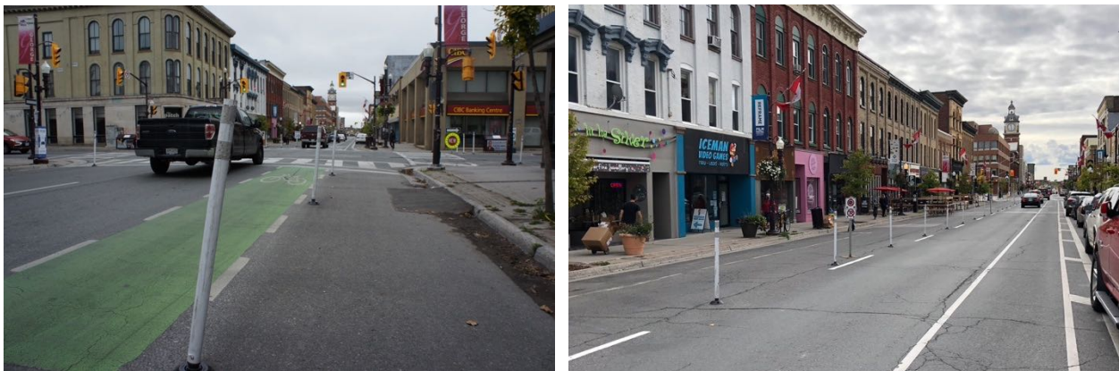
Figure 33. In many cases bike lanes were left on the roadway side of flexposts, unprotected from moving vehicle traffic.
