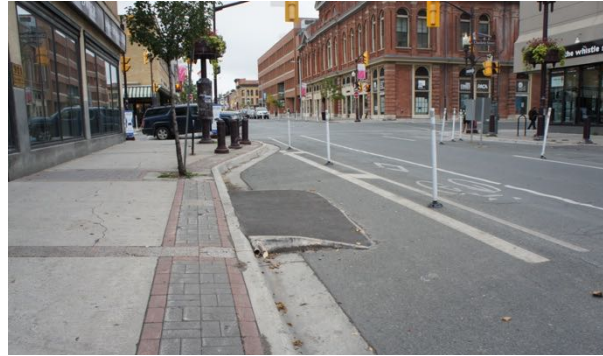
Figure 26. Patios blocking sidewalks created an accessibility issue if ramps were not provided regularly.
