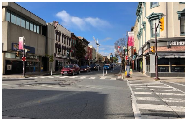
Figure 32. Intersections had unused, ambiguous space which can lead to potential safety concerns.
