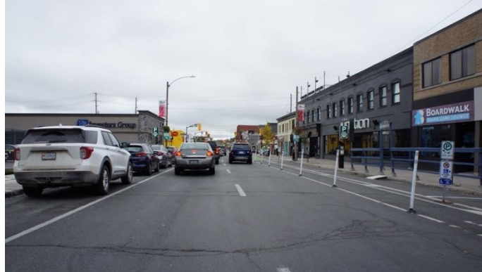
Figure 28. A parked vehicle obscures flexposts creating confusion about parking and travel lanes.
