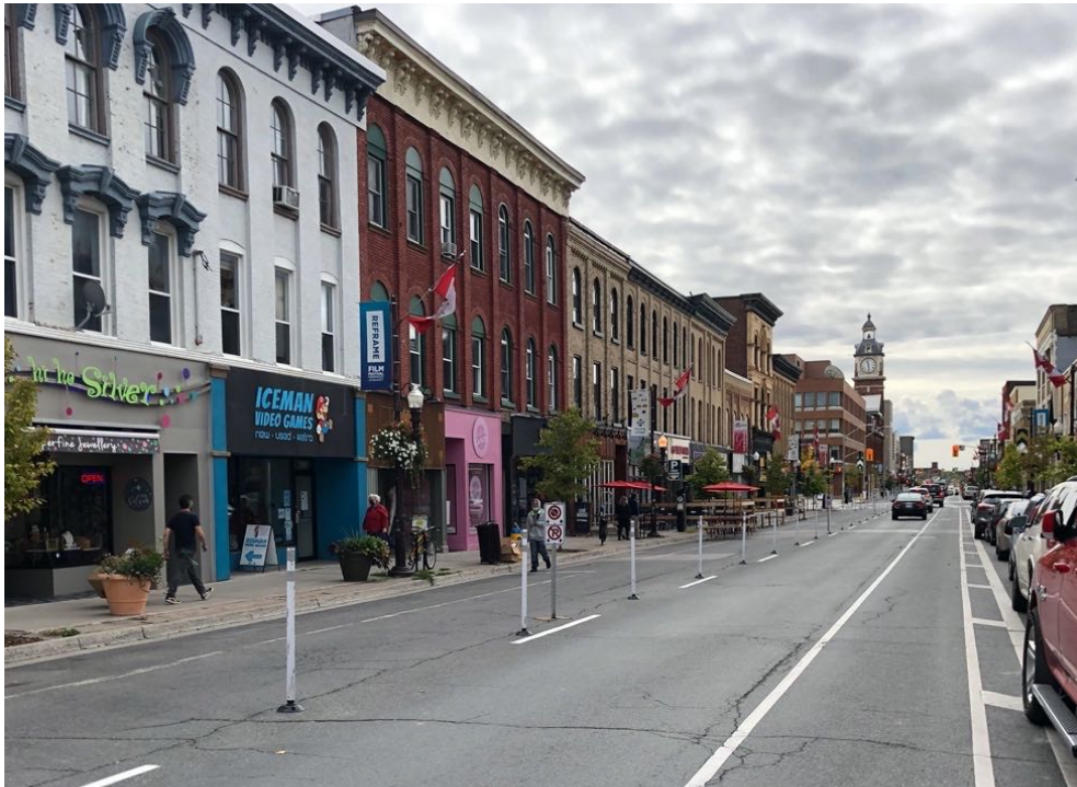
Figure 1. George Street in downtown Peterborough while the measures were in place.
