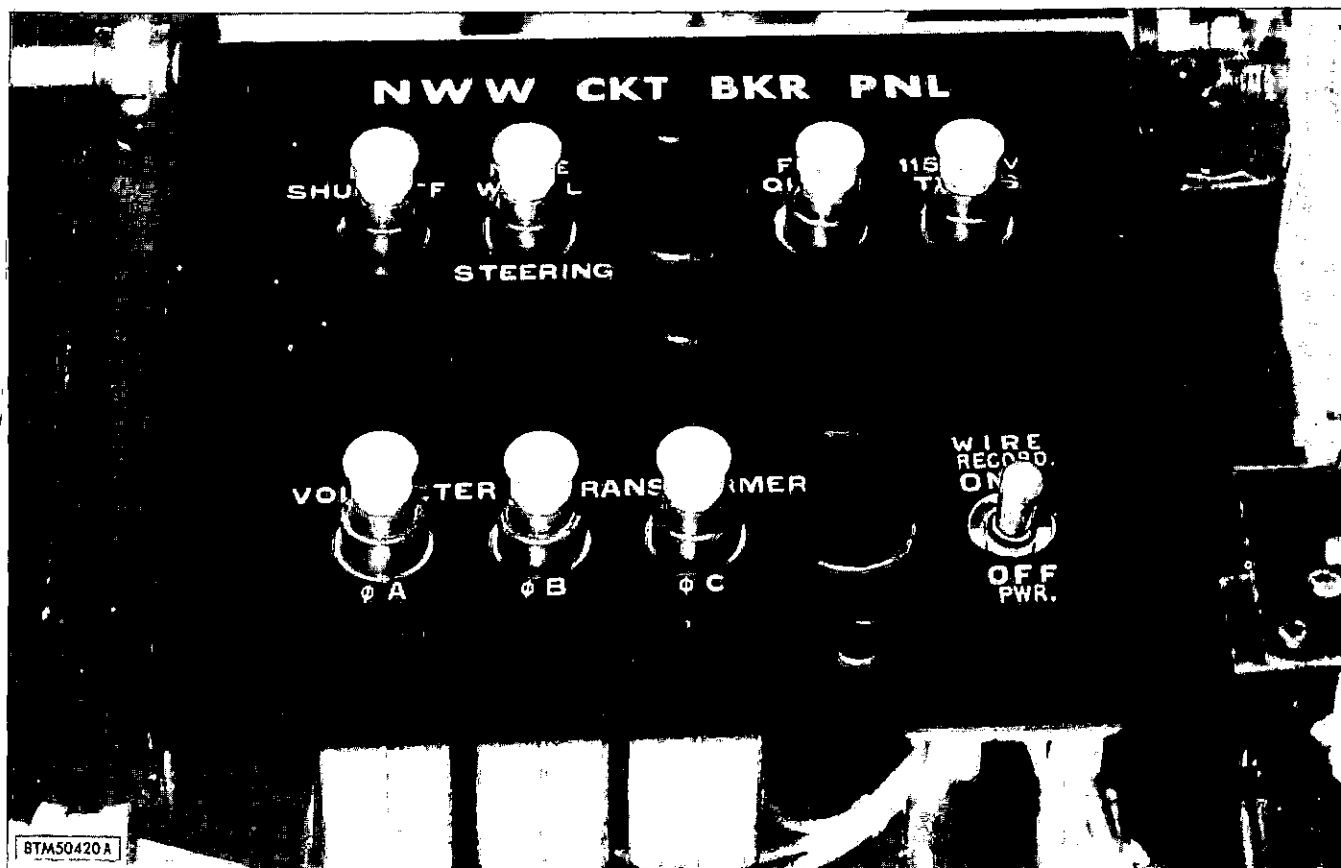
Figure 2-43. Nose Wheel Well Switch Panel
