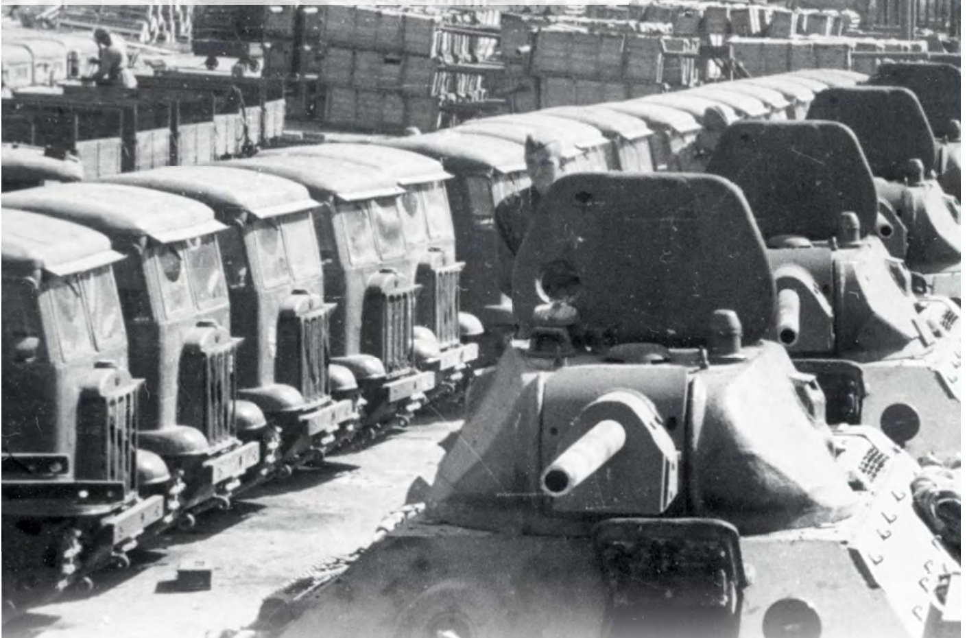
An STZ-3 in Red Army service. Note the all-steel road wheels and agricultural tracks
