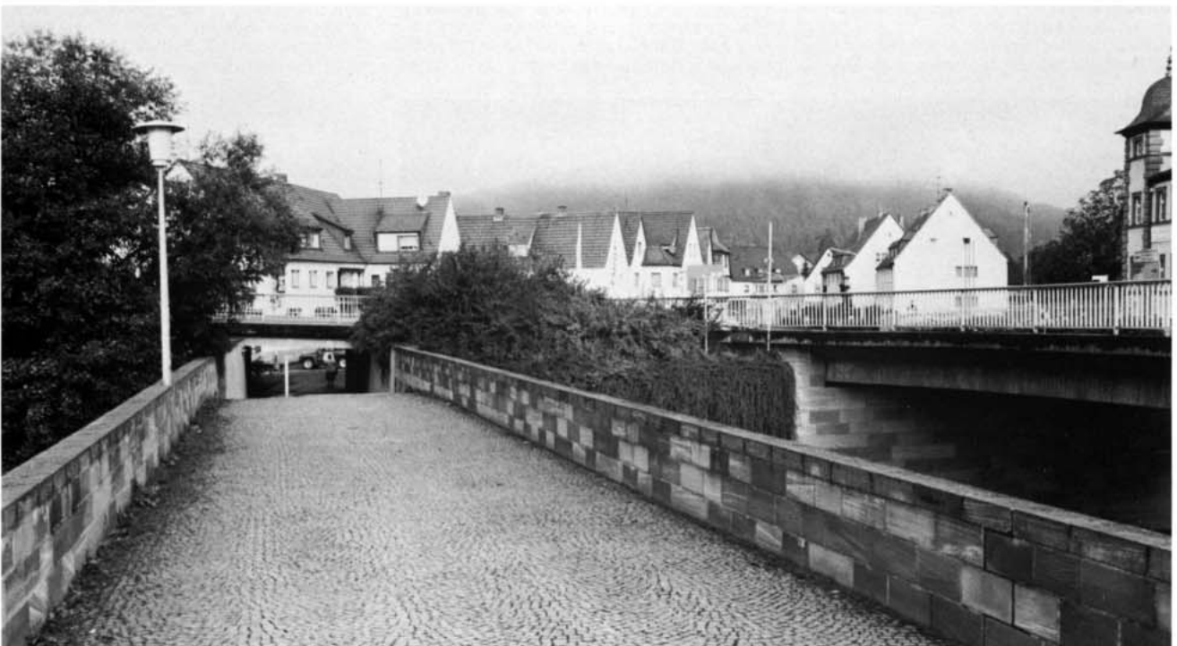
A new underpass now leads pedestrians into Frankfurter Strasse. A new bridge, visible on the right, now carries the road.
