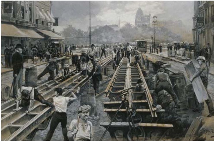
Laying Tracks at Union Square for a Railroad , an 1890 painting, depicts one of the era's many public works assisted by state and local governments.
