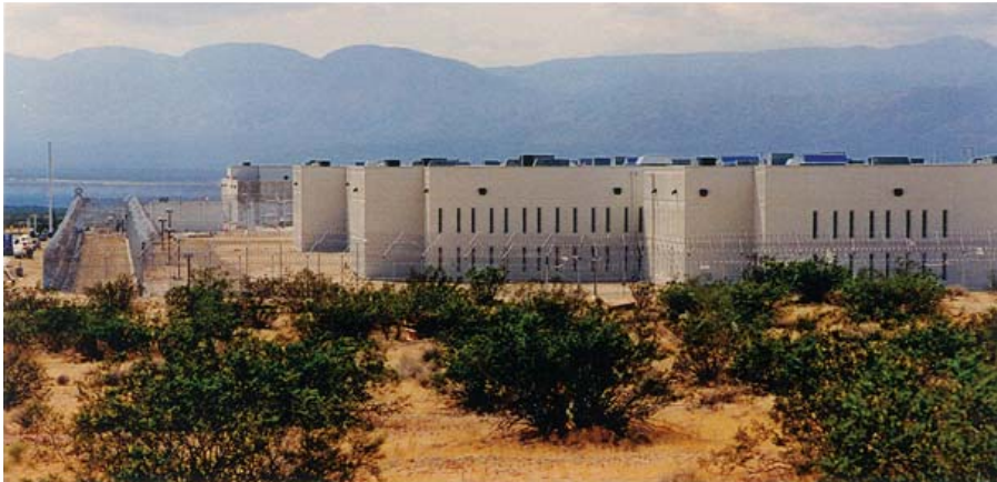
A private, for-profit, maximum-security prison under construction in 1999 in California City, in the Mohave Desert, illustrates the expansion of the “prison-industrial complex.”
