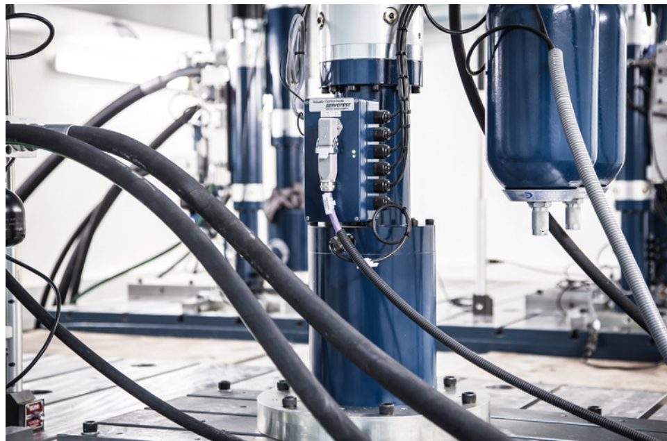
The control system allows the operation of each actuator as well as the synchronisation between them. Here a single Optostar fibre optic purple cable on the node box allows noise-immune digital data communication
