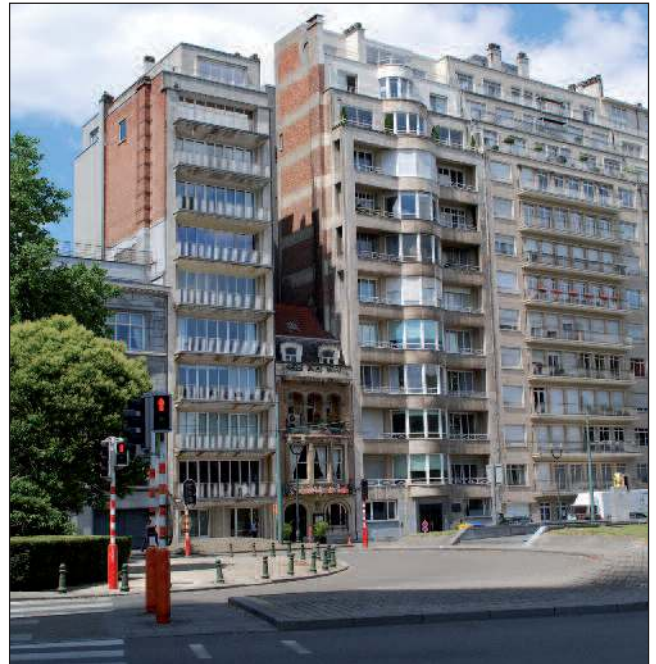
been built in 1936-37 so it was relatively new when the Sipo-SD moved in. Right: Known as the Résidence Belvédère, it remains unchanged but since the war similar tall apartment blocks have been built on either side.
