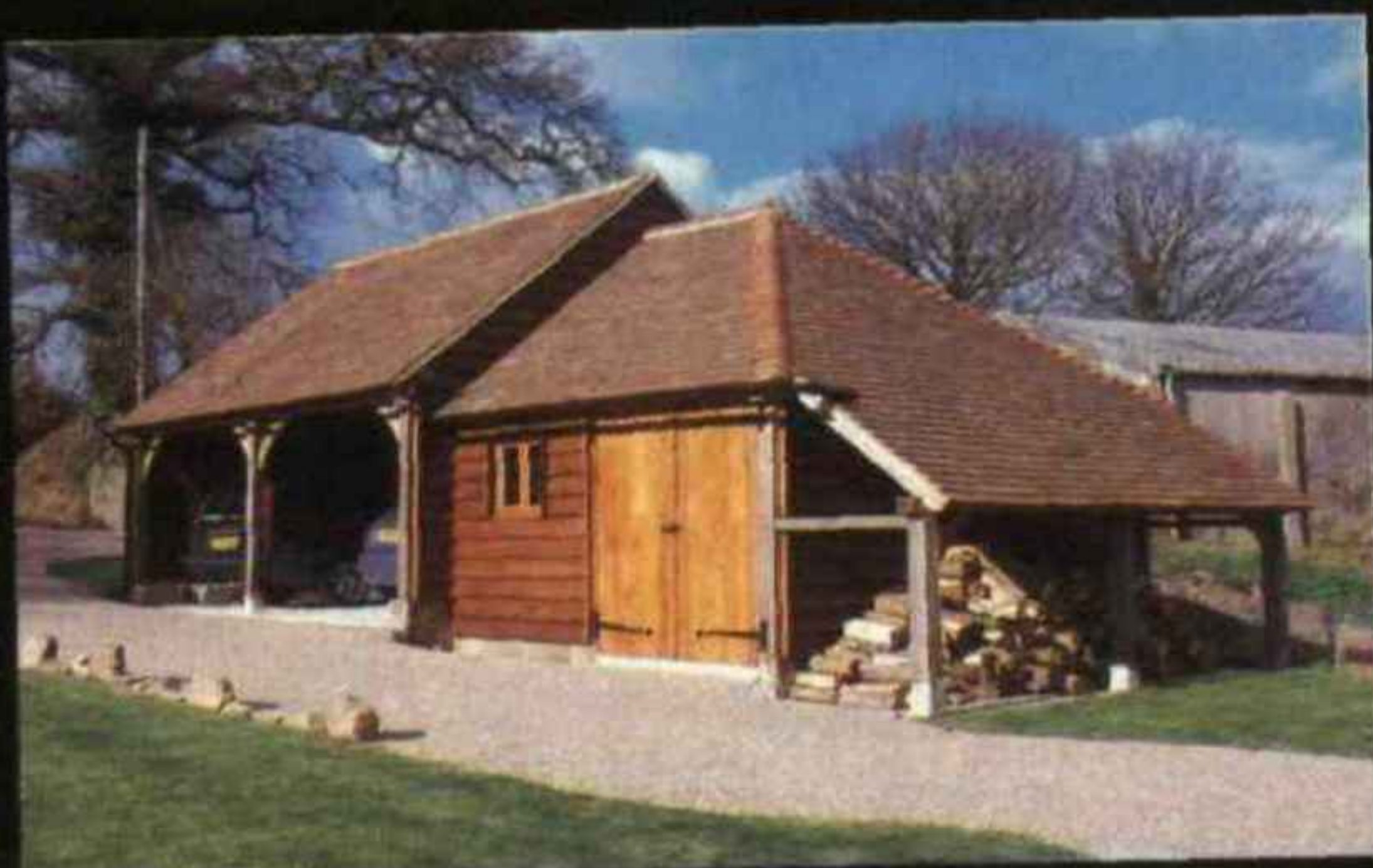
DOUBLE GARAGE, WORKSHOP & OPEN LOGSTORE
