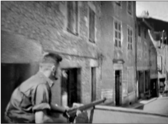
At midnight on June 8/9, the Vercors command issued Order No. 1 directing the civilian companies to move up to the plateau. Planned for months, the operation was swiftly executed using buses and lorries to bring up hundreds of men from nearby cities and communities. Left: A lorry carrying a
