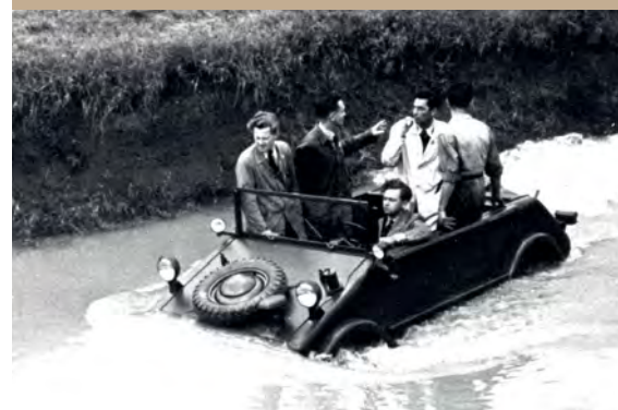
The end of September 1940 found Ferry Porsche at the wheel of the first Type 128 prototype as it surfed the Max Eyth Reservoir with a full complement aboard. Its Drauz-built body was doorless
