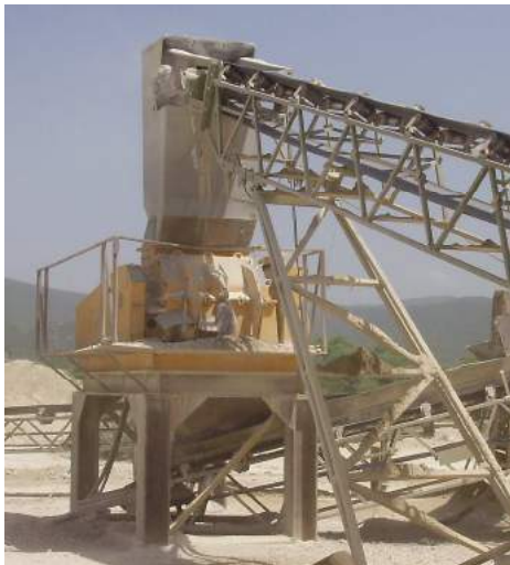
Figure 6. Stone crushing system
