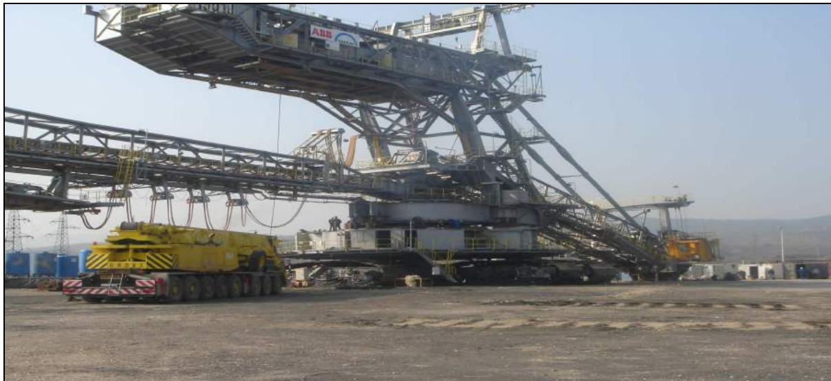
Figure 3. Photo, the settlement of excavator for repairing
