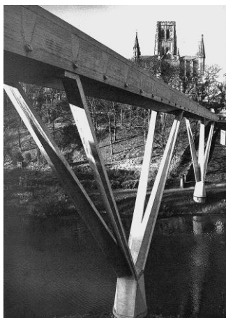
Figure 1. King's Gate Bridge (Source: Zokei 1996)
