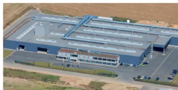
The family-owned German manufacturer is marking its 65th year in business with the opening of this new hi-tech plant in Wiethfeld
