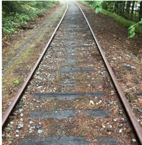
Figure 18: Typical Ballast Along the Corridor
