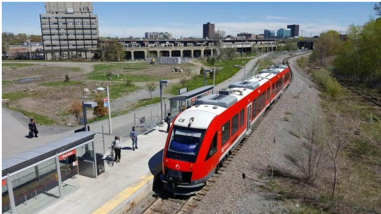
Figure 28: Comparator Station – Bayview, Trillium Line, Ottawa ( www.cbc.ca )
