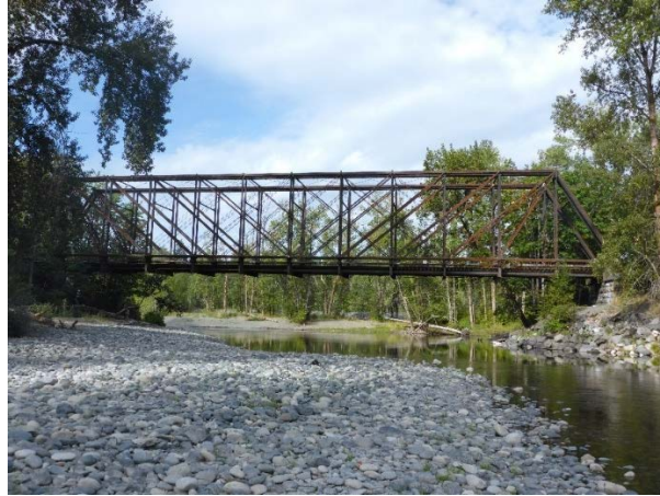
Figure 21: Cowichan River Bridge – mile 39.30
