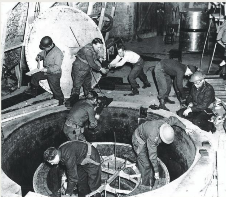
American soldiers dismantle the Nazis' experimental research reactor (left) at Haigerloch, Germany, in April 1945. The reactor featured a lattice design of metal uranium cubes (below). It was not until late in the war that the Allies were able to reliably assess just how close the Germans were to developing an atomic bomb.
