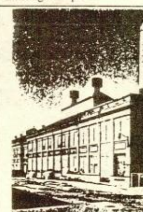
BUILDING 108, the Central Power Plant for the old Charlestown Navy Yard, will become office space as well as home to a banking facility and computer center. Boston Investment Development Company received tentative designation as developer of this parcel at the March 20th BRA Board meeting.
