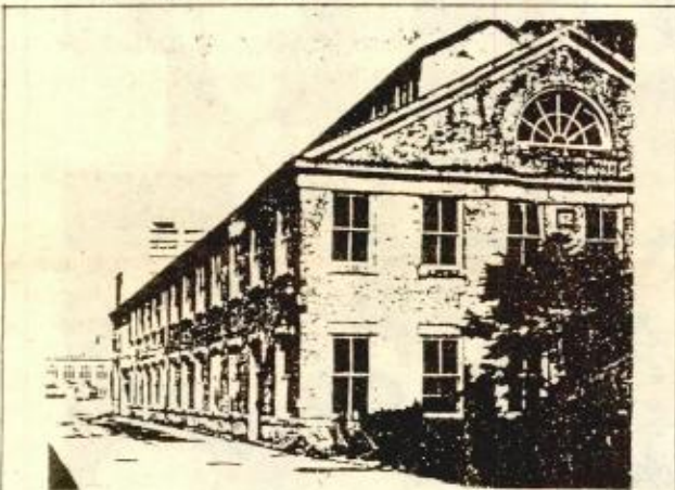
BUILDING 62, located in the Historic Monument Area of the Charlestown Navy Yard, was formerly utilized as the Ropewalk extension, test lab and "Hemp House." New Medico Associates has been awarded tentative designation by the BRA to rehabilitate the facility into office space.
