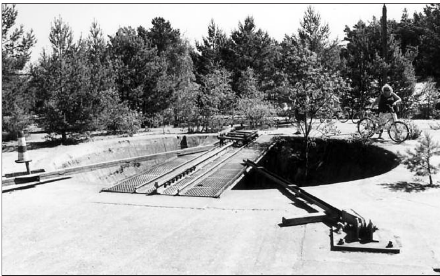
The best preserved part of the former Luftwaffe firing range is undoubtedly this concrete pit that was once the firing ramp for the Rheintochter anti-aircraft rocket. Developed — as the Rheinbote had been — by Rheinmetall-Borsig, this rocket could carry a 150kg warhead of high explosive up to 15000 metres (50,000 feet). Using optical tracking, the operator guided it by radio signals into a flight of enemy bombers at which point the warhead would be detonated by an acoustic proximity fuse. (K. Rogala)
