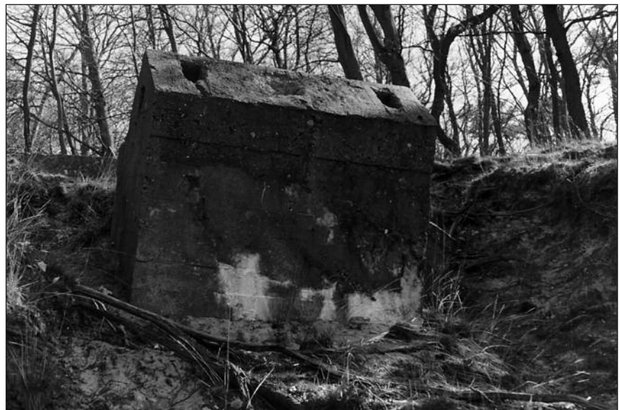
Left: In 1944, the Wollin area was German but now it lies in Poland and Misdroy has been renamed Miedzyzdroje. (Kalkofen is Wapnica and Lebbin Lubin.) Above: The HDP test gun was built on the side of a hill, with the lower part of the ramp standing directly on the ground (see top) and with large concrete supports to carry the upper part of the cannon. (A. Gilens)
