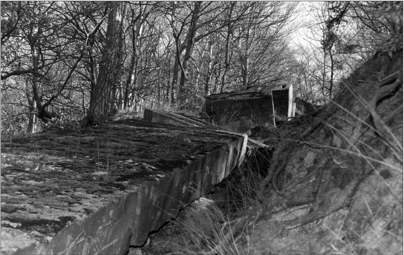
The bottom of the first ramp (see page 6) is now in the back garden of a private dwelling and the owner, Artur Jakisz, kindly allowed Alvin to take these pictures. Mr Jakisz recalled that the last pieces of metal and other non-concrete parts were
