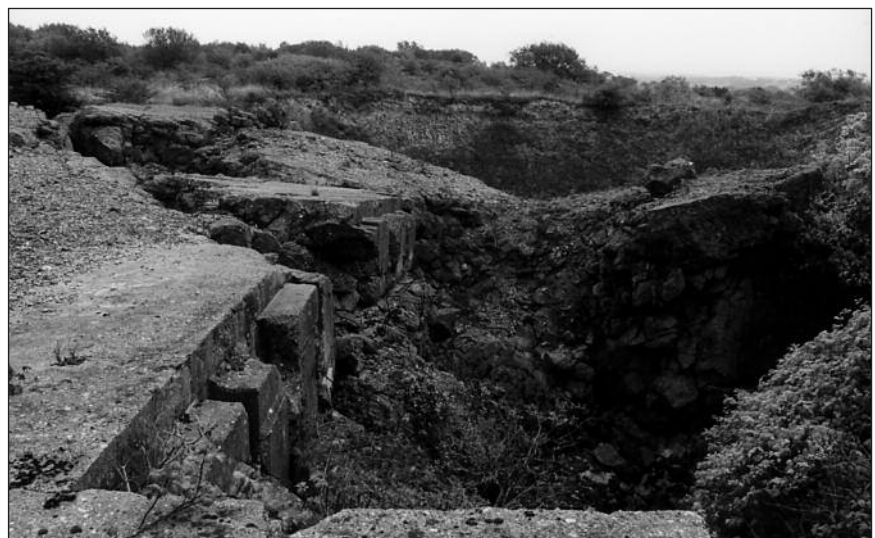
Our comparison shows a surviving corner at the top of shaft No. V. In the background, the crater of the Tallboy which clipped a corner of the concrete slab.
