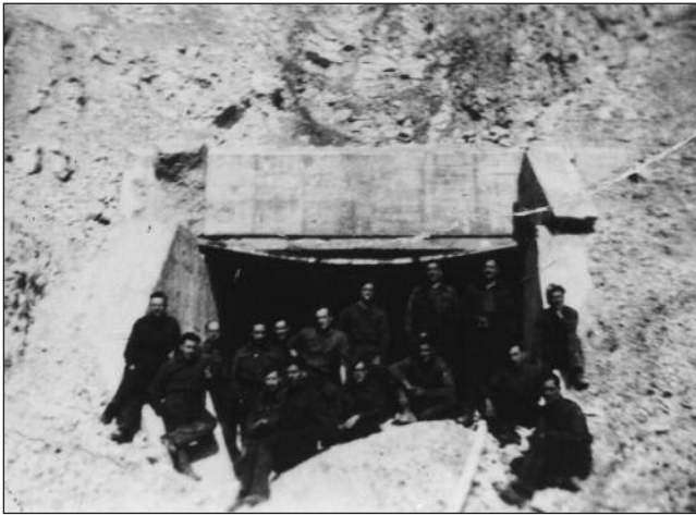
Left: This was the southern entrance of the railway tunnel as it appeared late in 1944 during the inspection by Colonel Sanders. Note the pipe bottom right, probably one being used to pump out flooded chambers. Colonel Sanders' mission was on site for four months and in his report dated February 21, 1945, he concluded that the installation could be repaired and pose a threat to London. It was therefore decided to destroy the underground facilities and Royal Engineers packed ten tons of explosives in the galleries. The resulting explosion on May 9 failed to close the entrances and a further 25 tons was blown at either end of the railway tunnel on May 14 (see After the Battle No. 6). Right: When in the early 1960s it was decided to use the abandoned tunnels for a mushroom farm, 30 metres of the hillside above the old southern railway entrance had to be removed to establish a safe access.
