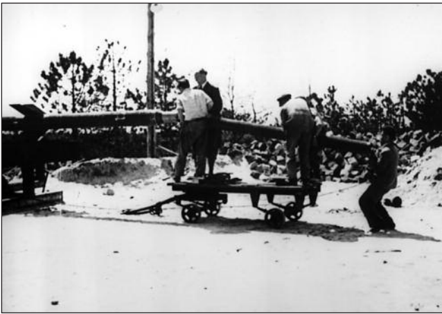
Left: With the third stage in place, technicians are seen here inserting the cylindrical guide which was the rear of the fourth stage. Obviously, the support equipment available at Leba was makeshift if not crude. The technical team seen at work in these pictures included military personnel from Versuchskom-
