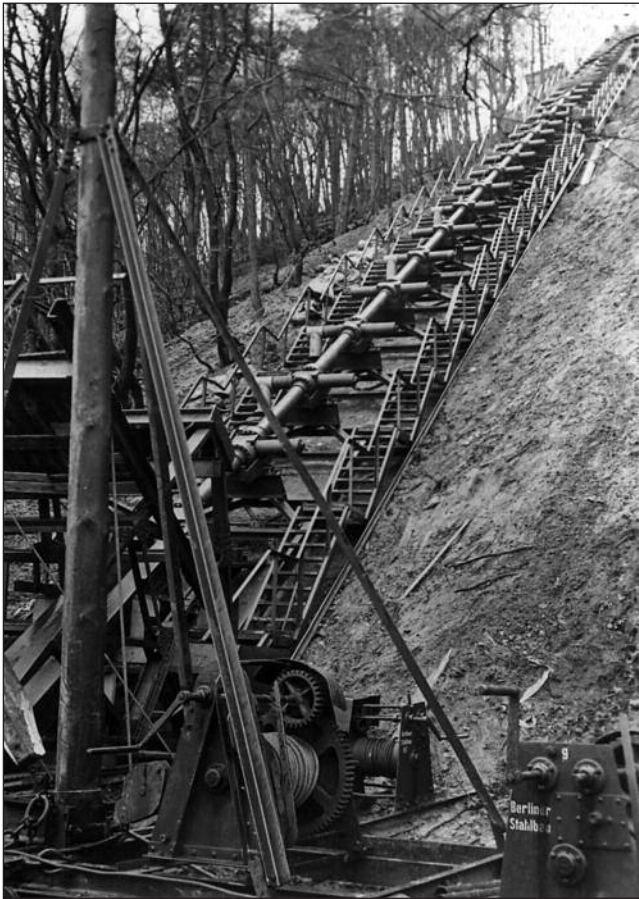
Left: Having attended a demonstration of the HDP at Misdroy, Generalmajor Dornberger wrote: 'An enormous number of gunners was required to service the weapon, standing on the staircases that ran to right and left sides of the barrel, and reloading the T-pieces with propellant charges between rounds'. (Bundesarchiv) Above: Alvin Gilens discovered this surviving ramp which still shows — as does the 1944 picture left — the long one-piece concrete slab which lay beneath it.
