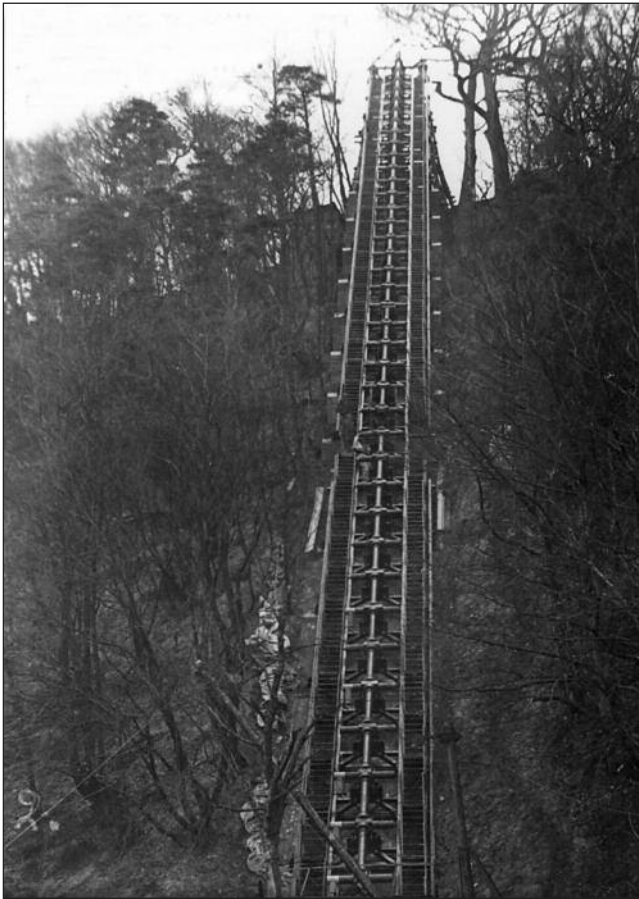
Left: Careful examination of the two pictures taken in 1944 proves that they actually show one and the same gun. (Bundesarchiv) Above: Two test guns were built at Misdroy and Alvin found out this second ramp 100 metres away from the first one shown opposite. The lower part of this ramp appears to have been built in a series of steps and not as a continuous concrete slab which indicates that this is not the same ramp shown in the two contemporary pictures. (A. Gilens)
