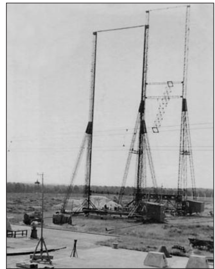
This device which had been installed to measure the speed of the missiles test-fired from Leba was probably also used for the Rheinbote trial launches. (The picture is now available as a postcard at the nearby village of Rabka.)
