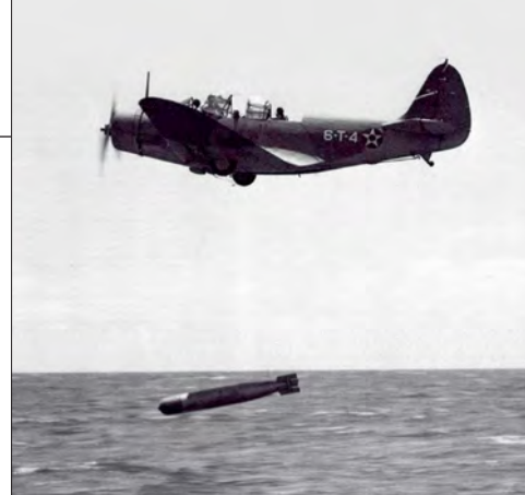
Above: A US Navy Douglas TBD-1 (BuNo 0325, 6-T-4) of VT-6 from the aircraft carrier USS Enterprise (CV-6) making a practice drop with a Mark 13 torpedo on 20 October 1941. TBD-1 0325 was destined to be the last surviving Devastator, being stricken on 30 November 1944 and subsequently scrapped.
