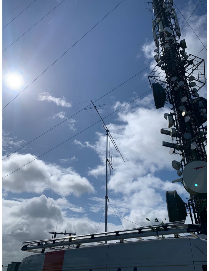
Our 2m horizontal and smaller 2m vertical beams next to the Cairn Hill mast
