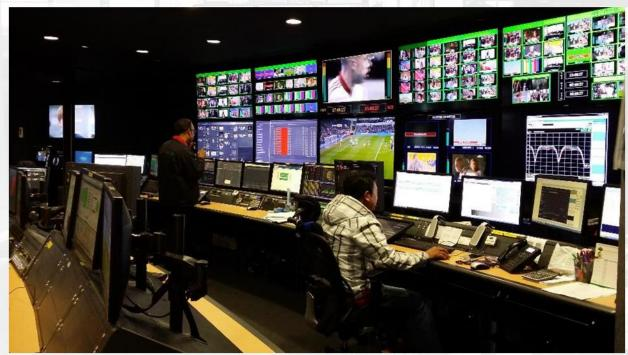
IDEAL Systems in Singapore designed, and built the new broadcast system and facility for GlobeCast Asia. This system has an initial capacity for 15 local playout channels and 20 turnaround channels headend, which are transmitted throughout Asia.
