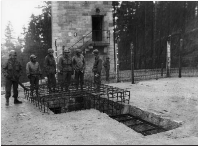
In the rear corner of the camp, next to one of the watch-towers, the Americans found a curious construction. In the autumn of 1944, with the number of inmates dying at the camp increasing rapidly, the SS had designed a method to efficiently move
