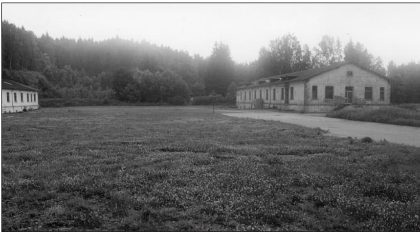
The kitchen and bath-house are today the only buildings surviving around the former roll-call square. For many years they were swallowed up by post-war factory workshops built around them and so were difficult to recognise. They emerged in their original state when the later buildings were removed in 2000.
