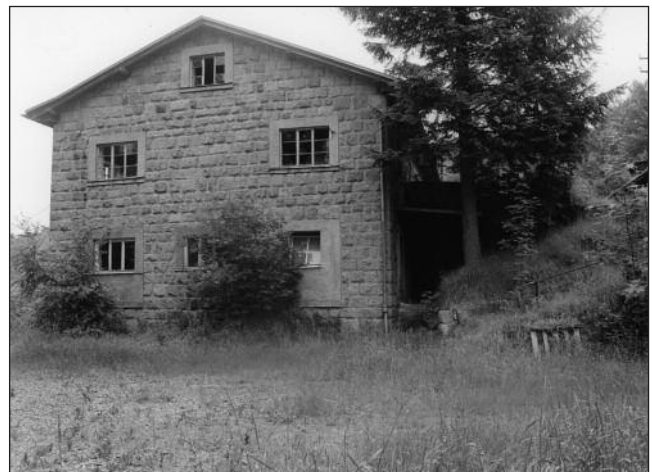
Our comparison was taken closer in, with our back against the wall of the quarry's transformer station.
