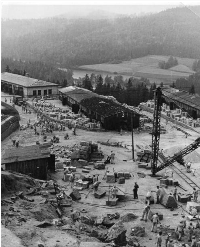
Above: Before 1940 the men had to quarry by hand with nothing more sophisticated than picks and jack-hammers. Later heavier equipment such as cranes became available. The granite was sold for use in the Reich's prestigious building projects, the residue being used for autobahn construction. The building on the left is the quarry's garage [D]. (NIOD) Top right: The garage can be seen among the trees on the left. Part of the shed on the extreme right also survives.
