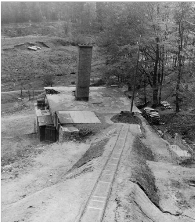
. . . on which a small trolley car ran down narrow-gauge rails straight onto the roof of the crematorium. The trolley could be used to transport corpses and also carry fuel for firing the
