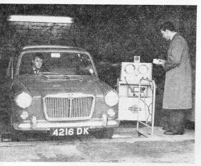
AN M.G. 1100 makes use of the Crypton Walker Road Load Dynamometer at B.R.T. Developments.
