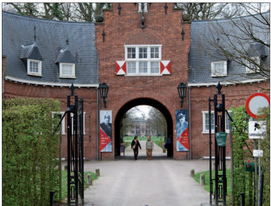
The gatehouse and main entrance on Langbroekerweg remain unchanged.
