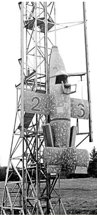
ABOVE: Fully fuelled and ready to fly, M23 hangs from its launch ramp awaiting only its pilot. Sieber's padded head rest, attached to the cockpit hatch lid, can clearly be seen.
