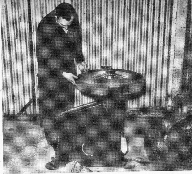
Tug Wilson balancing a Borrani light-alloy racing wheel and Avon tyre.
