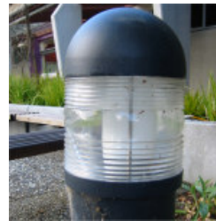
Look for alternatives if you can't find a real glass lens. This is an appropriate size security light fixed beside a footpath.
