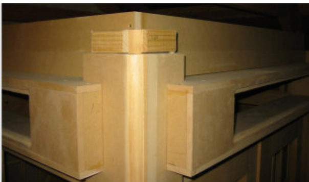
Step 1 reaches up level with the top of the post, then the post cap sits on top, rising halfway up the height of the second step. This might vary depending on your design.
