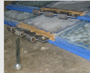
Half-hinges and a loose pin are excellent for taking the windows out of the Box.
