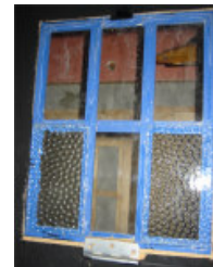
When complete, I held the windows to the door using a hinge at the bottom and Velcro at the top. You might choose to simply screw them to the back of the doors/walls.
