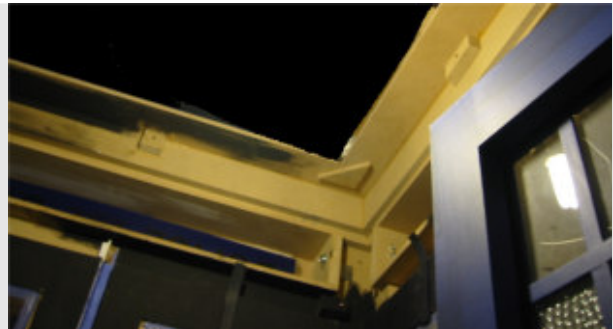
Internally, the first few steps were a very simple construction. Simply a square frame initially of the total height of the first 2 steps. After gluing and screwing together, this is surrounded on the outside by parts comprising the thinner first step which are glued to the outside lower edges. The top platform is almost a 2-D sheet made from 4 panels cut with 45 degree corners. These are slightly shorter than the total size of the step so that they will sit inside the frame. It is glued in place and then reinforced with corner supports and a few blocks along their length to add strength. Remember the next section of roof will be sitting on this platform later.
