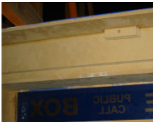
Small blocks on the inside help to keep the platform in shape and at the right height so that it can support the upper roof.
