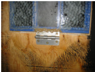
A lower hinge allows these windows to open inwards and the choice of another "loose-pin" hinge means that the windows are very easily removed.
