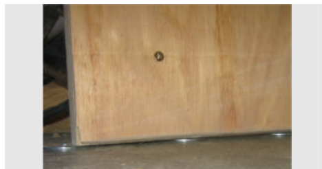
An old carpenter's trick apparently – put a couple of coins under the door when you hang it - this means that it won't grind over or into the base/floor/carpet whenever you open your doors, while giving it a flat surface to rest on during your hanging efforts..
