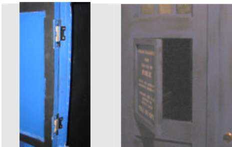
Here, the panel has hinges attached to the side, set into a slight recess that I chiselled out. The rear half has been routed so that a panel can be pushed in from behind.
