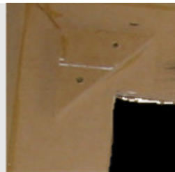
A piece of scrap wood is screwed underneath each corner of the platform which holds it all together since glue alone would flex and break quickly.
