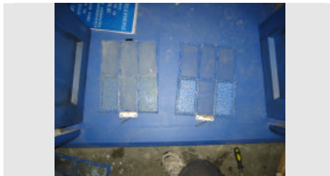
Be sure to plan out which windows goes where. Once the hinges are attached to the frame you can line up the window and screw the other half of the hinge to the doors/walls – but I found that every windows was attached in a slightly different spot so they are now assigned their own unique locations.
