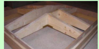
Joining the framework together could be done a number of ways, with brackets or by cutting slots so that the pieces mate tightly.
