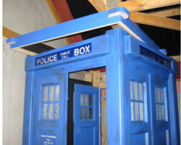
This section of the roof simply drops into place over the box structure and sits on the back of the sign-boxes. It drops down so that the first step is at the same height as the corner posts, and then the post caps sit on top of that level.
