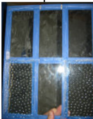
The "window" is made up from Perspex cut to a T-shape which covers the back of the top and middle-lower frames.
