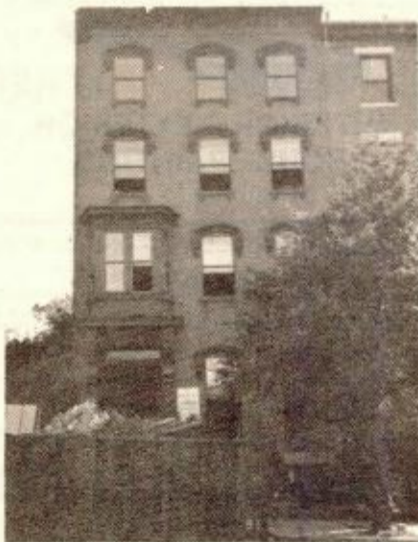
Possibly the most luxurious Condominiums in the town, now under construction with City and harbor views. Come see our plans. Prices range from $112,000 to $137,000
