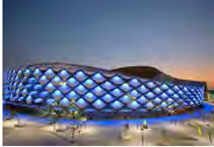
Hazza Bin Zayed Stadium, Abu Dhabi
