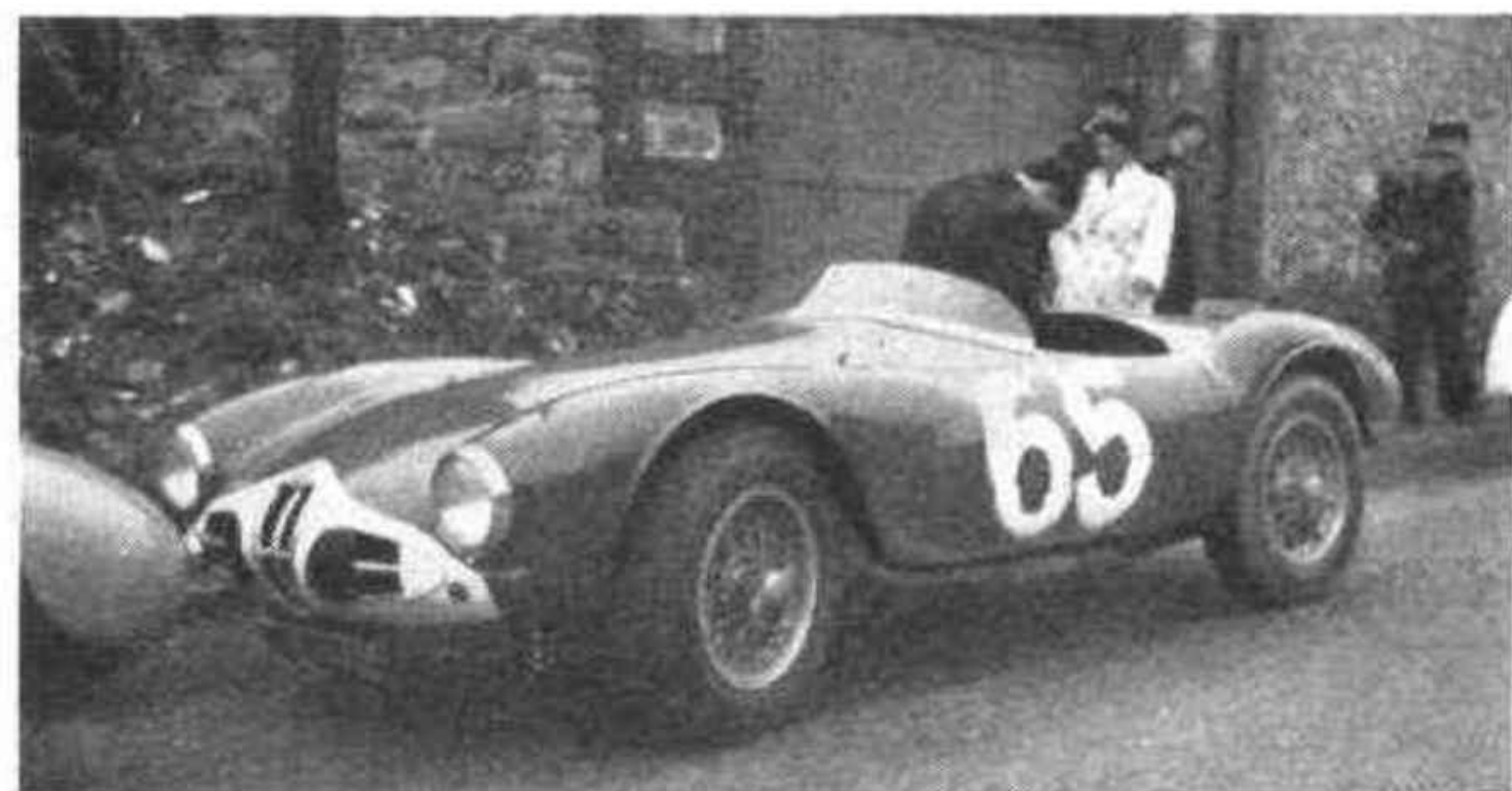
DISCO-VOLANTE.—The special Alfa-Romeo of the Swiss driver Ducrey. Using the same type of engine as the 1900 model, and many of the mechanical components of the production car, it proved to be a very rapid 2-litre.
