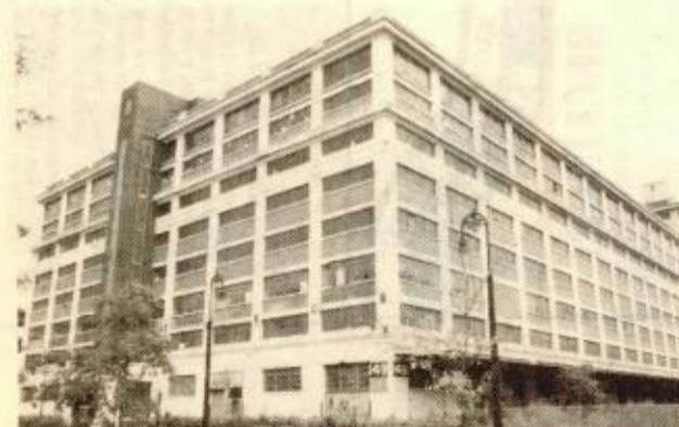
BUILDING 149 could become a Communication Center which is what Mayor White thinks will allow the Navy Yard to blossom into a prosperous business area. Behind Building 149 is a similar building which will be converted into a parking garage.
