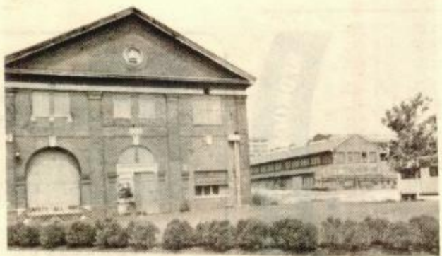
BUILDING 103 (left) will be rehabilitated with Section 8 funding and made accessible to elderly and handicapped. To the left is a section of Building 104 which will also be converted into 50 more low income homes for the elderly.
