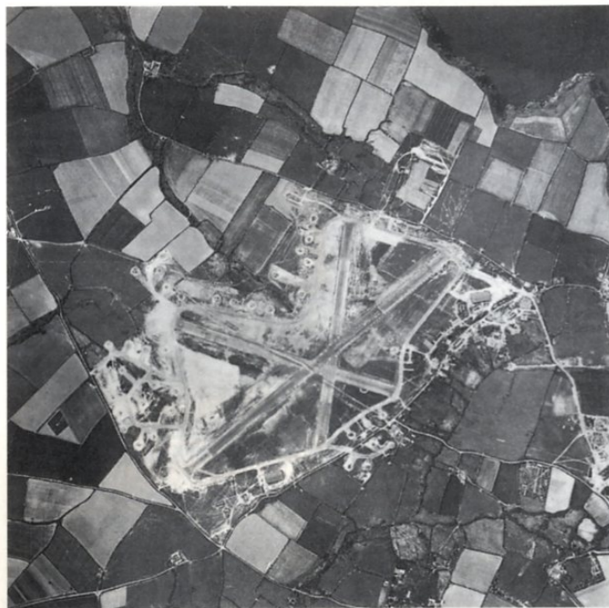
Talbenny in May 1944 looks almost like a building site, although most of the dispersal areas have occupants.
