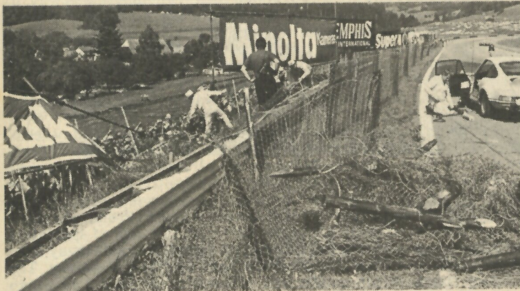
The path to destruction (top). Note the large wooden (and heavy) catch fence posts which have, along with the fencing, acted as a launching ramp. Also note the ridiculously low Armco barrier and the drop beyond. The wrecked March (below) with the roll over hoop and forward facing struts straddling the advertising scaffolding which probably inflicted Donohue's head injuries on impact. The aftermath (bottom).
