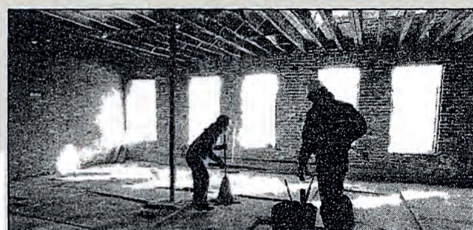
Sweat-equity renovation work under way in tenement at 66 Avenue C.
