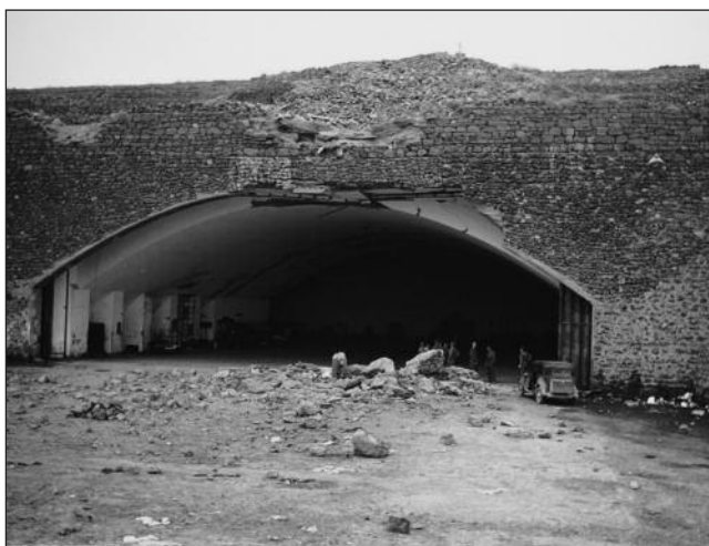
Left: One of the two entrances of the underground hangar, pictured after the Italian surrender (note the damage on the rooftop caused by an Allied bomb). Designed by Pierluigi Nervi, a well-known architect of the Fascist era, the underground hall was partly dug out from the side of a hill but most of its protec-
