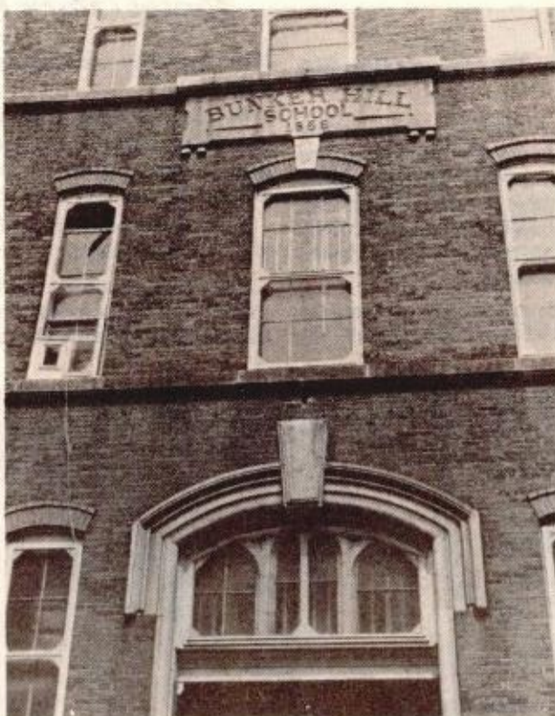
THE FORMER BUNKER HILL SCHOOL at the corner of Baldwin and Bunker Hill Streets will be the focus of a meeting on Wednesday evening, February 15th as proposals are presented to the community for re-use of this 118 year old structure.
