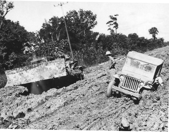
Above: A Caterpillar D7 of Co A, 1880th Aviation Engineer Battalion, is coming to the rescue of a Jeep bogged down between Makum Junction and Digboi (US NARA).
