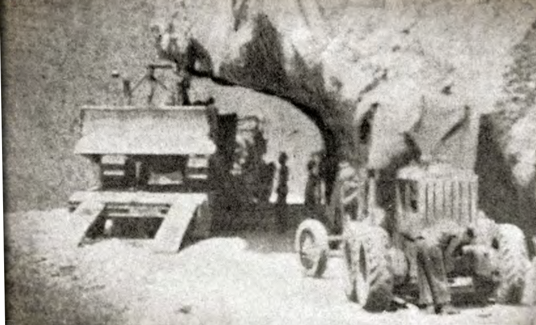
Above and left: Passing underneath a low-ceiling passage bored through the rock demanded the unloading of each equipment from their trailers (1880th Aviation Engineer Battalion).
