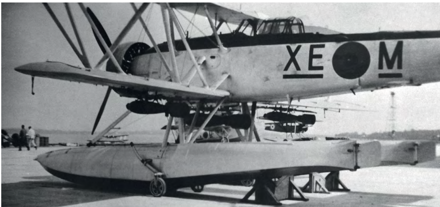
Shark III 524/XE-M of No 6 (BR) Squadron, loaded with 250lb bombs beneath the wings and a 500lb bomb under the fuselage. The larger, squarer rudders of the Boeing-built MkIII's floats compared with their Blackburn equivalents can be seen to advantage. MATTHEW WILLIS COLLECTION
