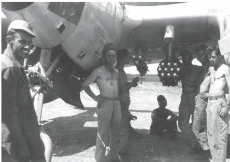
At that time, a new added weapon to the P-38 was rockets carried in pods of 10 and what looks to be a group of three to the left of the pod. (Photo courtesy of Jack Watson via Warren Thompson)
